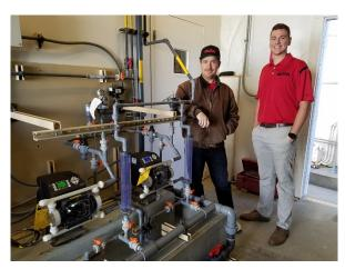
**Result:** The MD3 succeeded in pumping the gas-forming chemical in the high pressure application and eliminated vapor lock. The pumps injected 12.5 to 16% of sodium hypochlorite at the rate of 5-7GPH at 80-120Psi. The MD3 pumps maintained an accurate and continuous flow, providing smooth chemical dosing and eliminating the need for a pulsation dampener.
